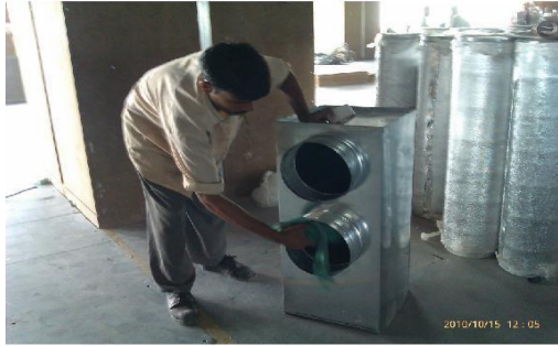
Cleaning Prior To Installation
